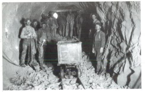
Men dug out a tunnel under the mountains to divert water from the Strawberry River while the dam was being built.
